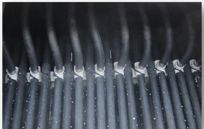
Those hoses are almost the only components we change in prevention every 7 years.
